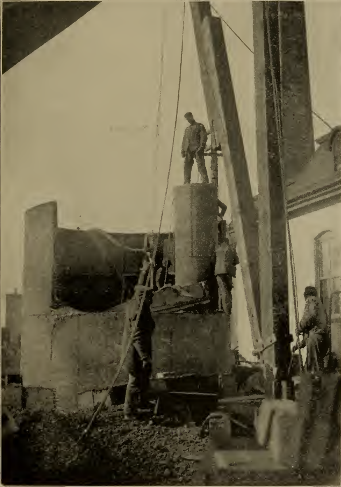
SINKING THE CAISSON—ROCKFORD, ILLINOIS.
